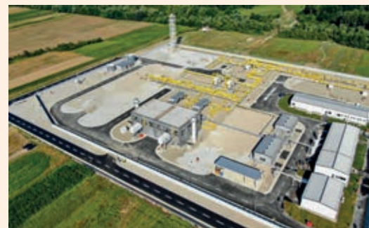
Transgaz's Bibesti compressor station.
